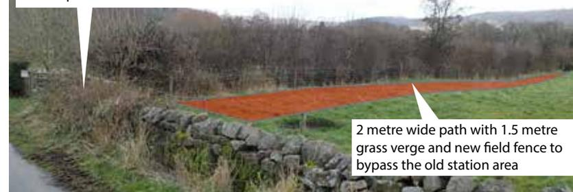
2 metre wide path with 1.5 metre grass verge and new field fence to bypass the old station area
